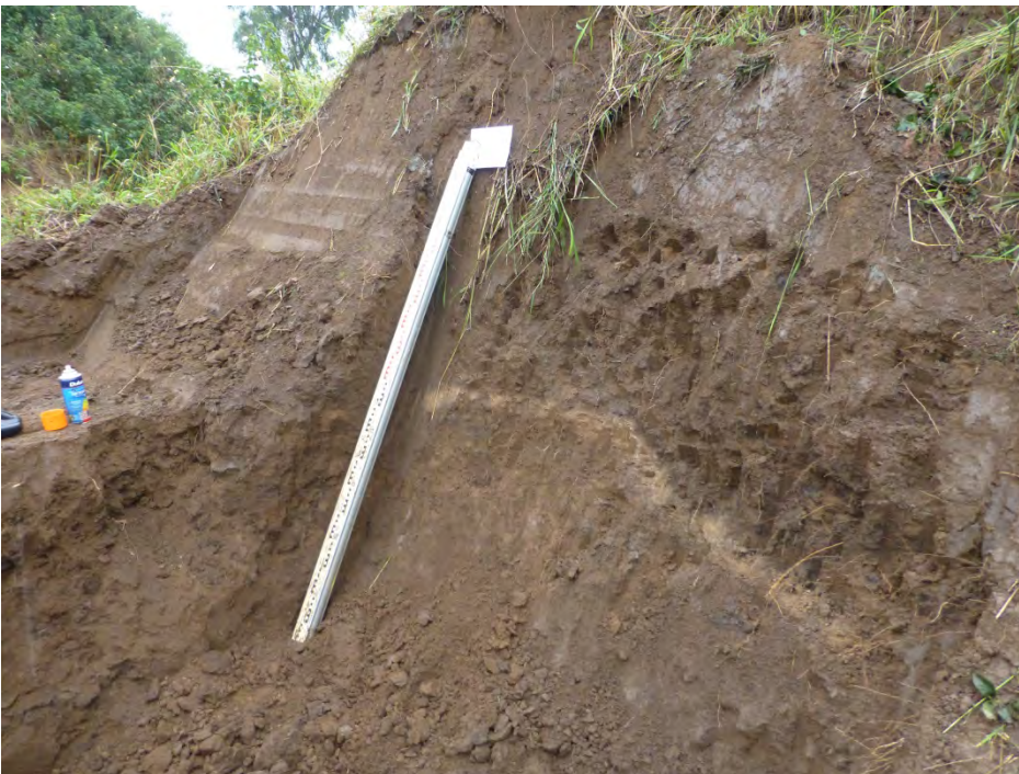
Photograph D64 – TP125 – North
