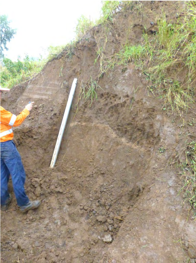
Photograph D63 – TP125 – North
