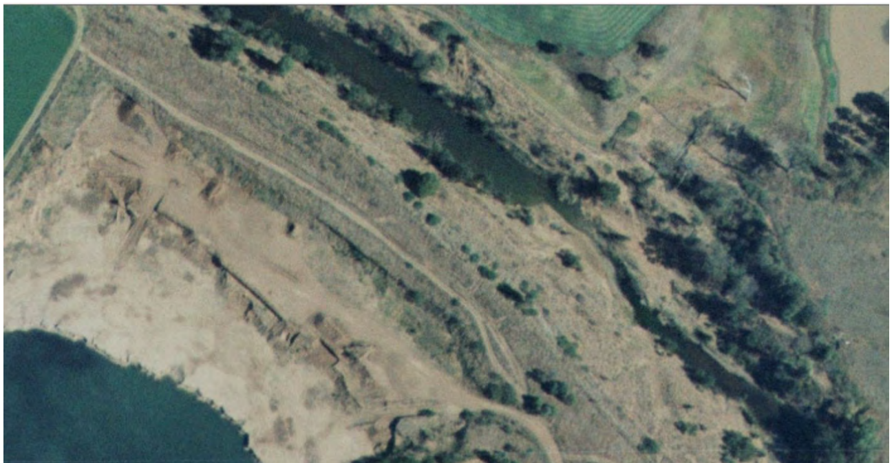
Plate 31b Enlargement of 1997 air photo showing western levee – note no bunds either side of access track
