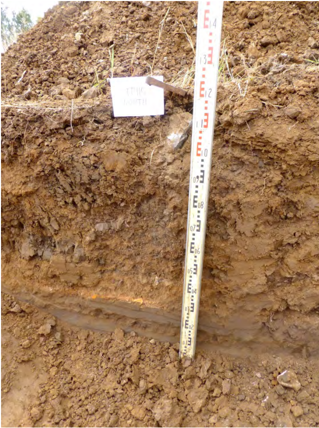
Photograph D44 – TP115 – North
