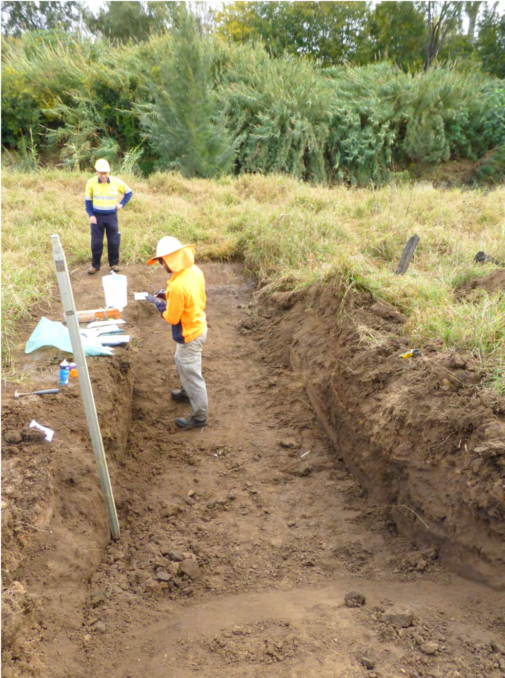
Photograph D5 – TP101 – General view.
