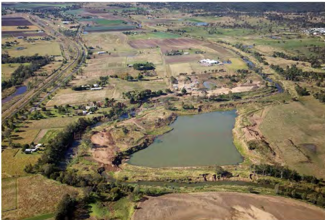
Aerial photo 2011 post-flood, looking east from the quarry and showing the remains of the northern wall around the quarry being demolished. Grantham town is in the top left of the photo.
