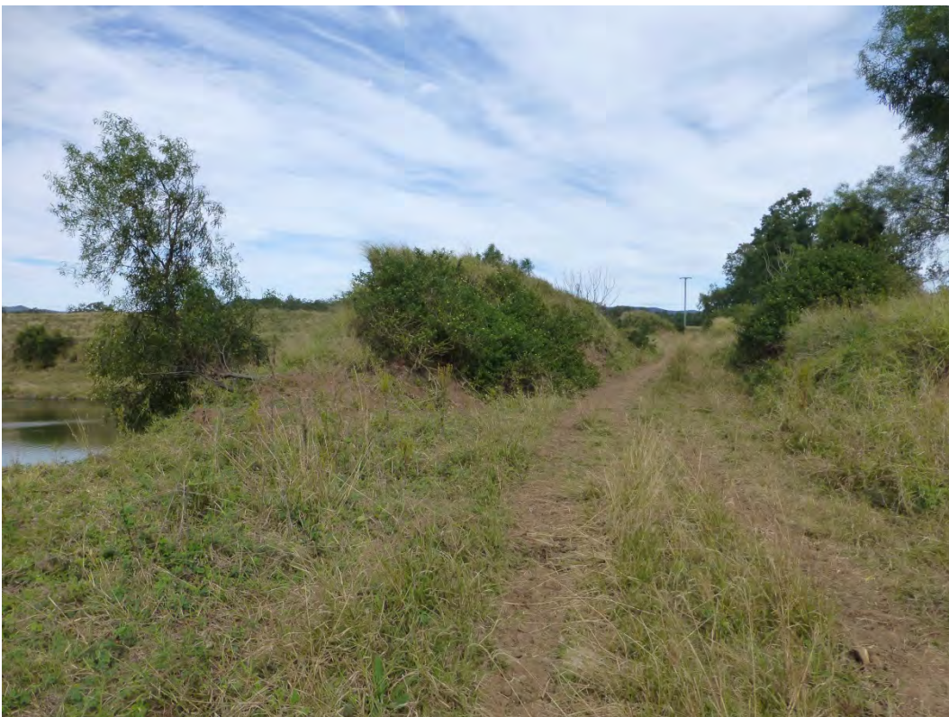
Photograph B4: Grantham Quarry – Track along Western levee – view towards South.
