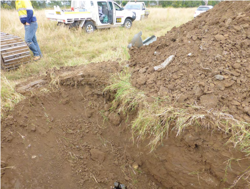
Photograph D46 – TP116 – Backfilling breach
