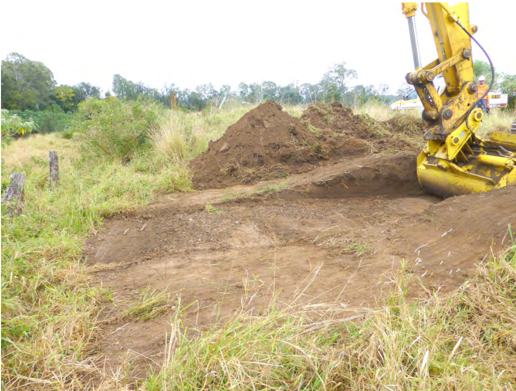
Photograph D38 – TP114 - Excavation in progress
