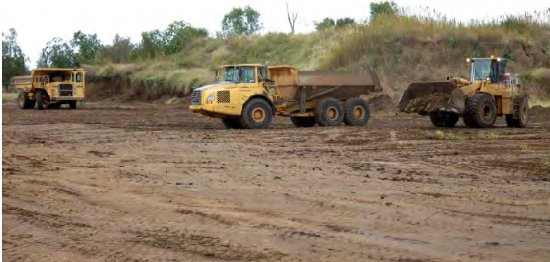
Heavy equipment demolishing part of the remaining earthen wall on the northern side of the Grantham quarry.
