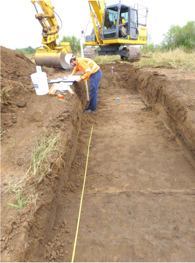
Photograph D42 – TP114 – General view of trench looking East.
