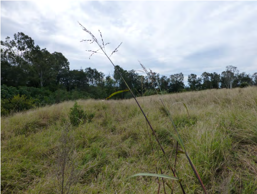
Photograph B3: Grantham Quarry – View along Western levee bank showing terrace.
