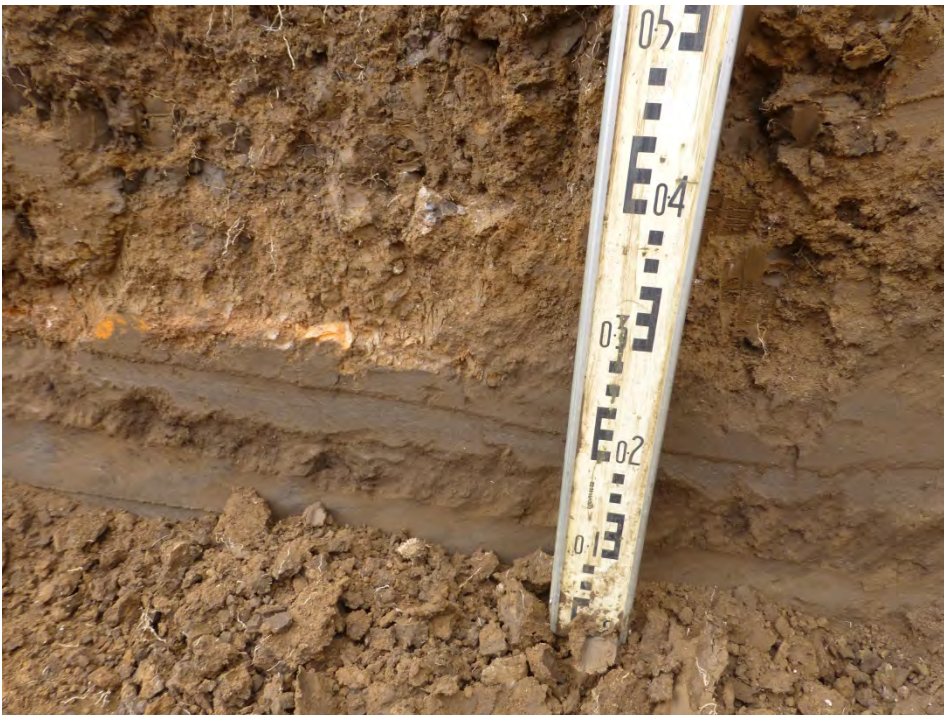
Photograph D45 – TP115 – Details of fill contact.
