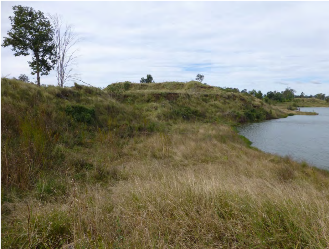
Photograph B1: Grantham Quarry – View from main breach towards East.
