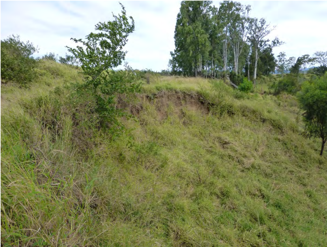
Photograph B7: Grantham Quarry – Erosion of Western side of levee from 2011 flood event.
