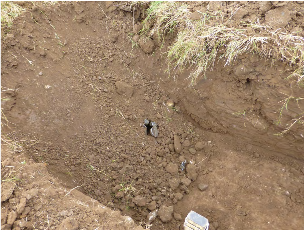
Photograph D47 – TP116 – Backfilling breach
